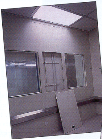
Figure 3B. Postcap utility chase runs between pre-fabricated steel panels to provide ready access for modifications or repair.
